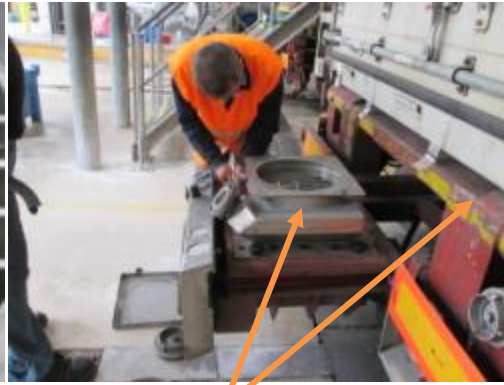
General lack of inspection eg not clean see loose product on chassis frame
