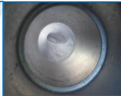
Inside of Rotary Valve outlet
