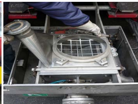
Fitting top plate on rotary valve
